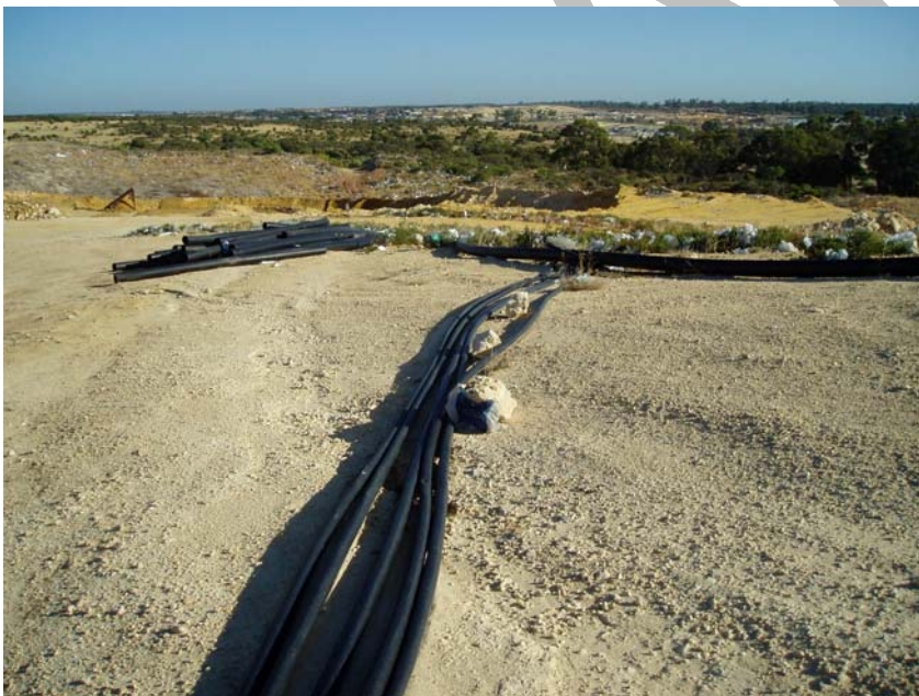
Figure 5: View from waste disposal site toward Clarkson showing landfill gas irrigation lines
