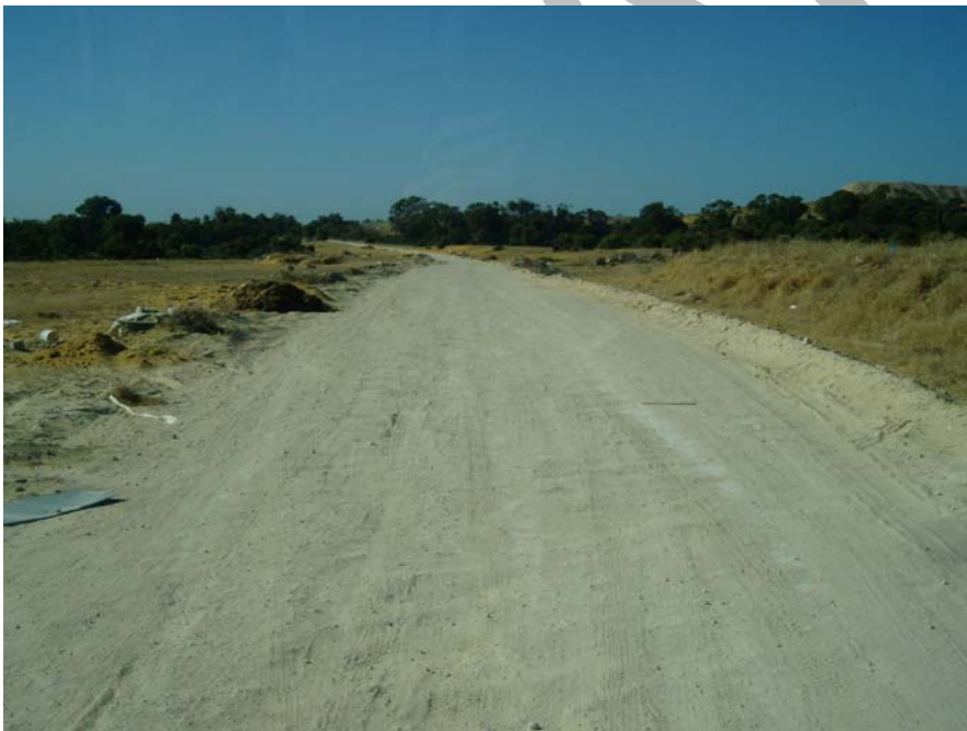
Figure 9: Connolly Drive extension -limestone stage
