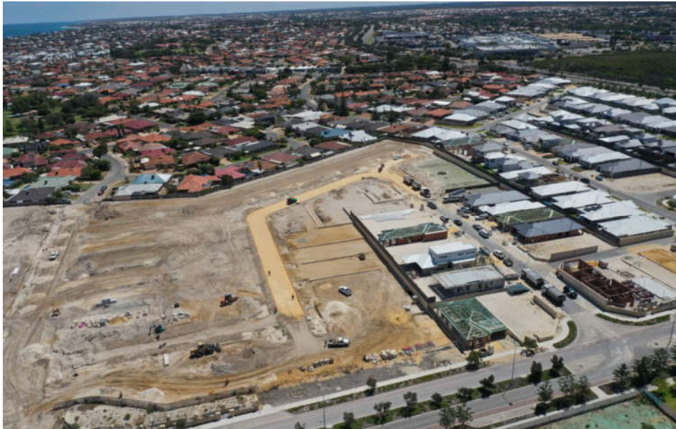
Construction of Stages 27B and 30 in progress
