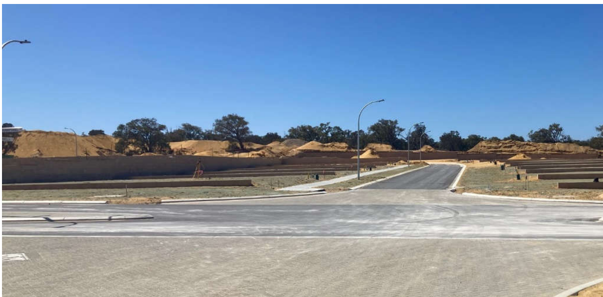
Completed Stage 38 Civil Works
