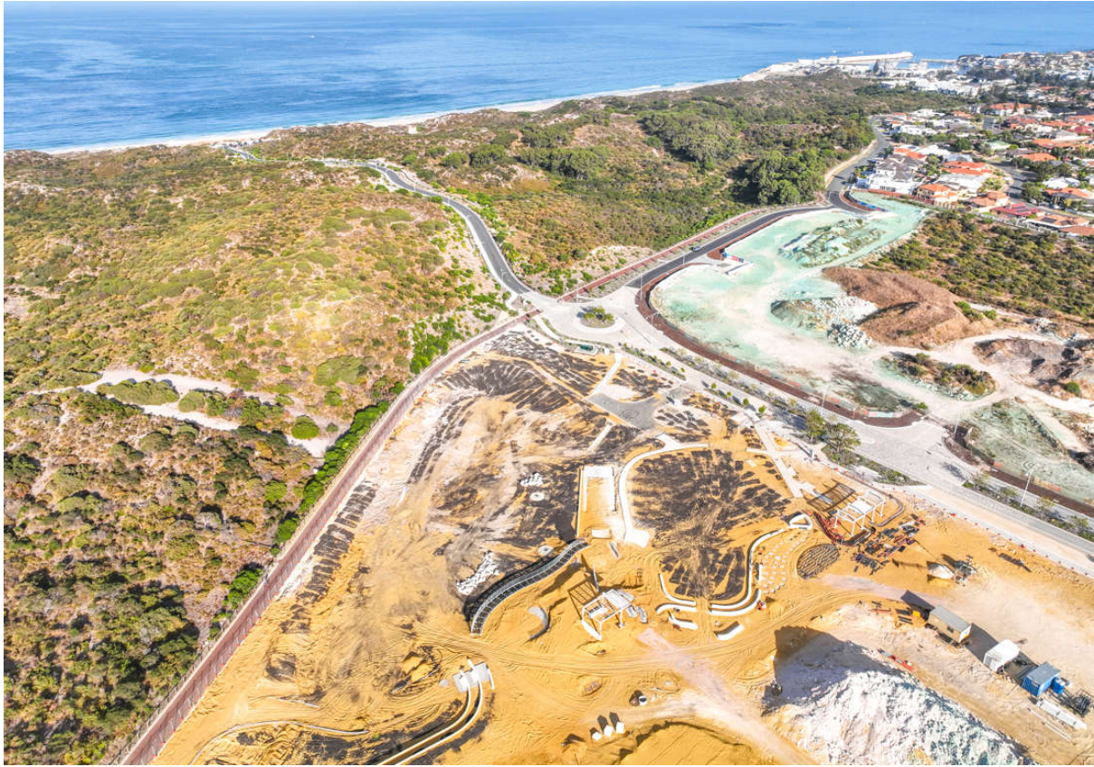
Foreshore Park under construction
