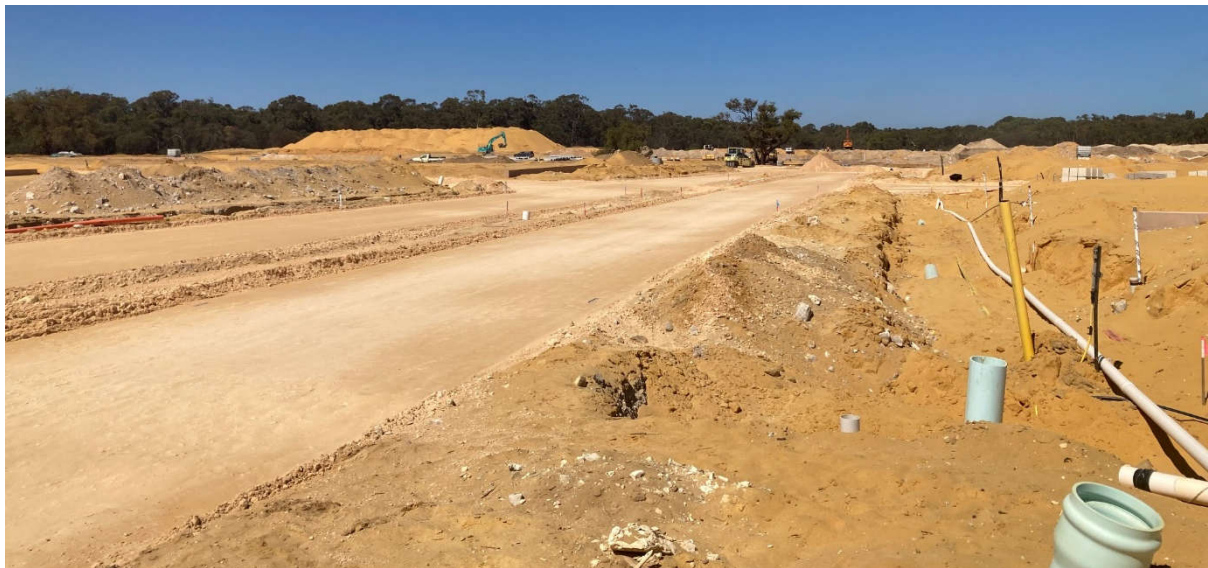
Stage 39 (in foreground) and Stage 41 (in background) Civil Works in progress
